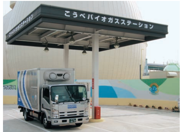
Bio gas station
