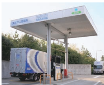
Home-use natural gas filling station (Chiyoda Station)
