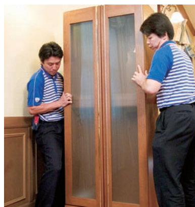
Installation by a sales driver and staff member
